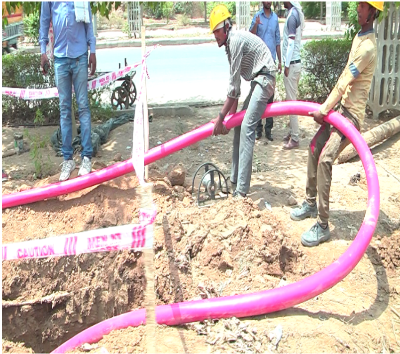
Helpers pulling cable from the drum
