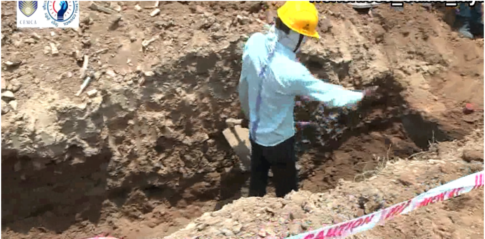
Extra digging for XLPE joint
