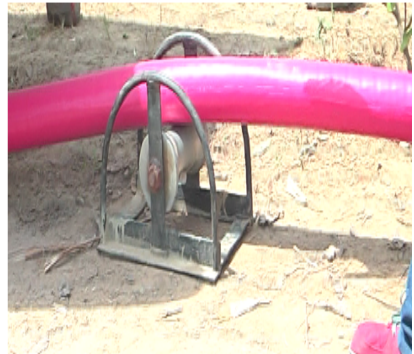
Rollers through which the cable passes
