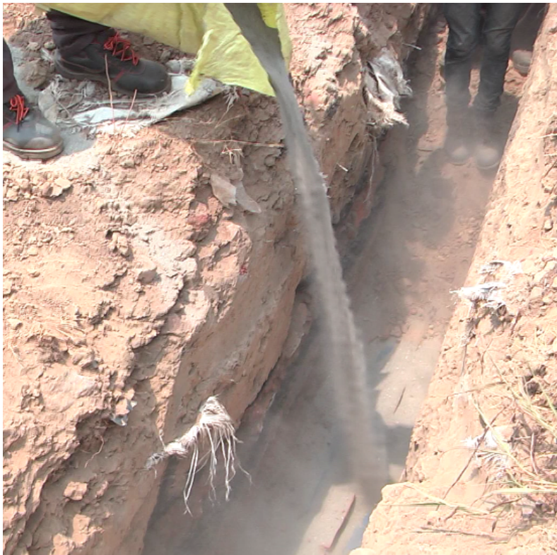
The trench being filled with soil
