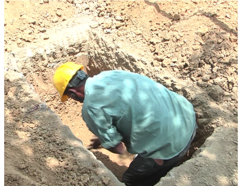
Digging a pit for laying trenchless cable
