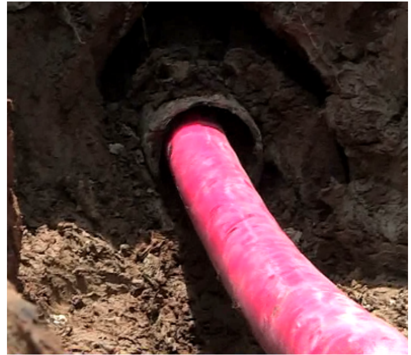
Cable going inside the pipe
