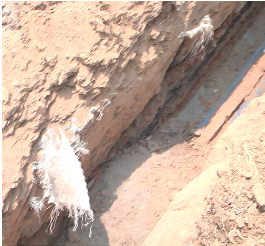
Excavated trench for double circuit
