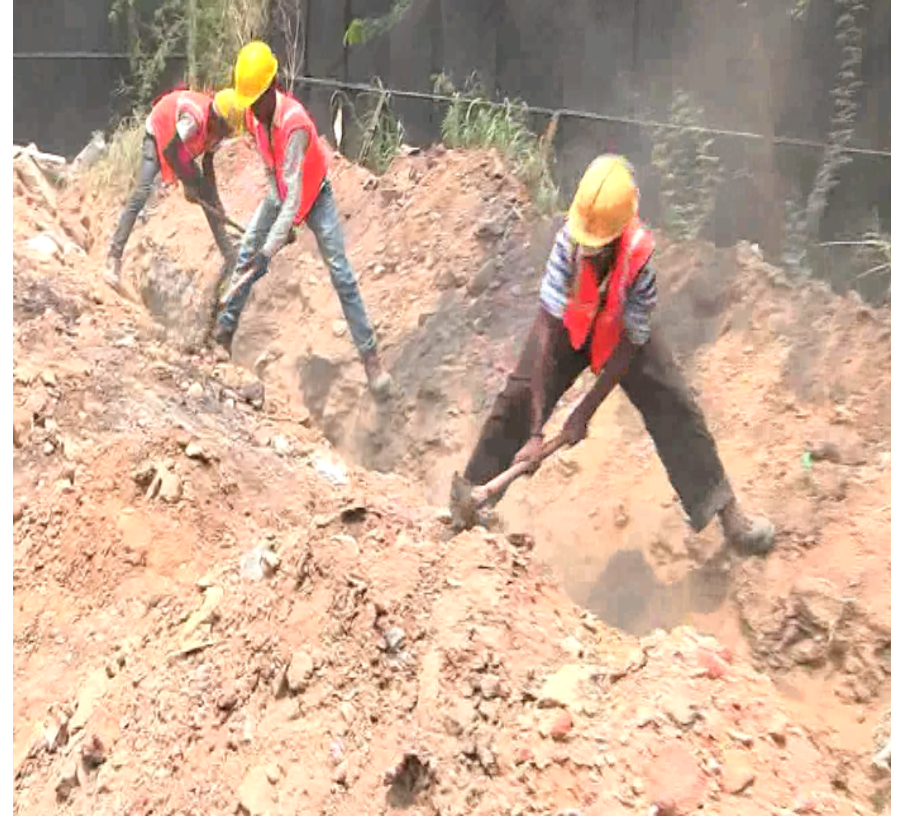
Filling the trench with hard soil
