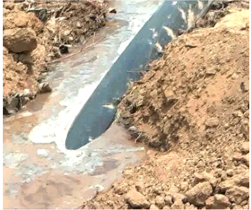
Insertion of HDPE pipe through bore
