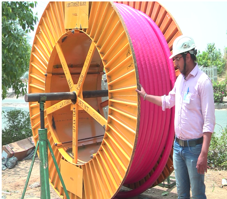
Cable attached to the drum jack
