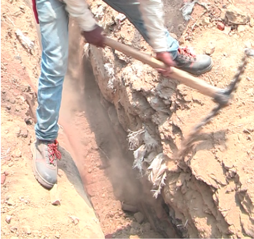
Filling the trench with soft soil first
